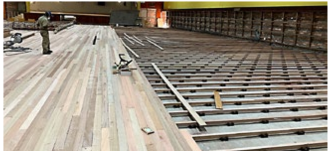
A new raised sports floor being laid on Instacradle rubber cradles, produced from recycled old truck tyres
