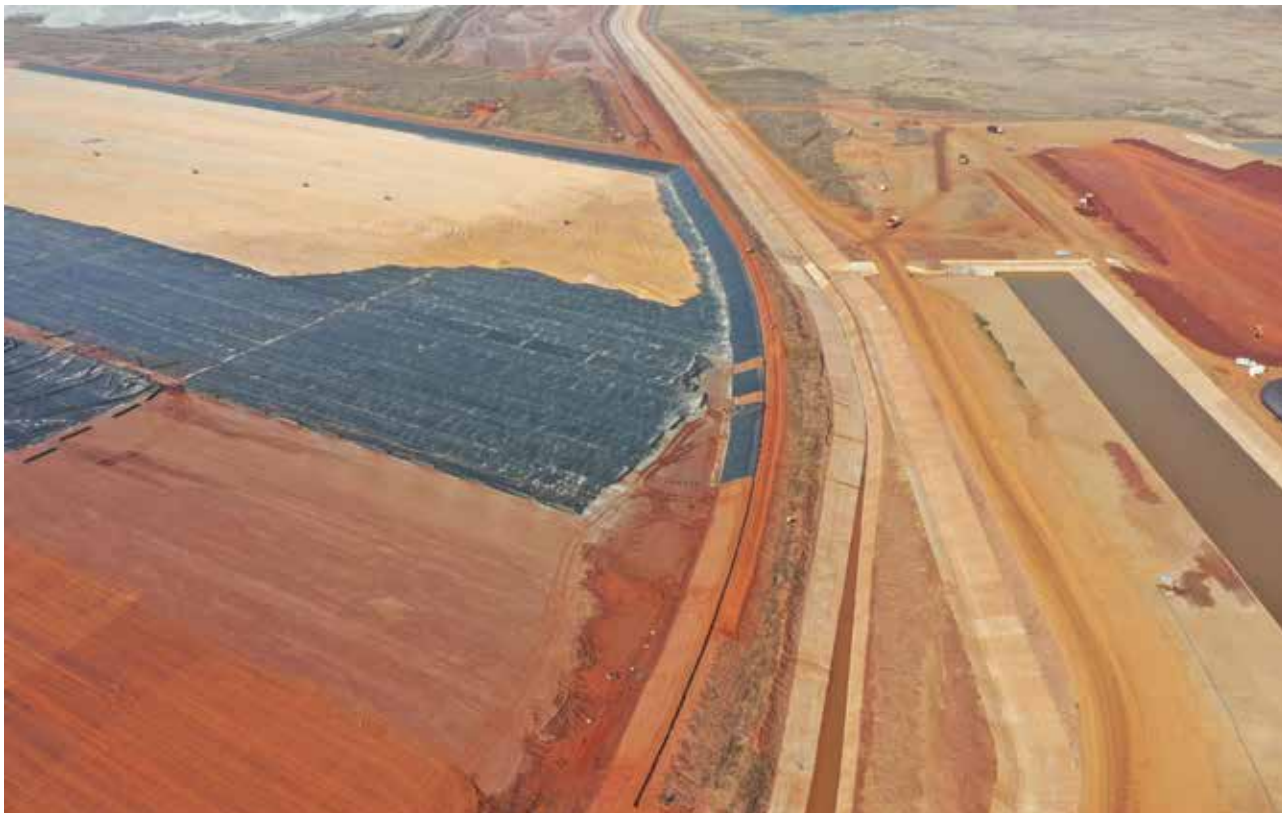
(Above): Two HDPE-lined earth dams hold clean water, while two similar dams will hold polluted water.
